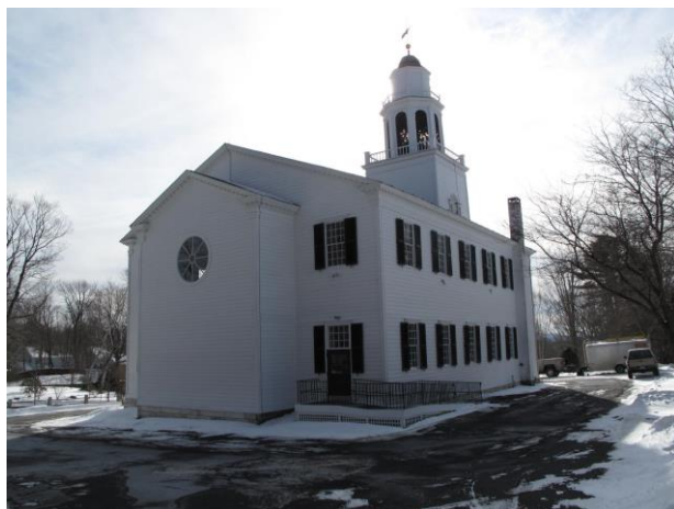
View from North Side Parking Lot
